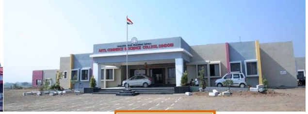
New College Building
