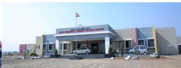
New College Building
