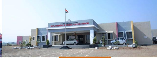
New College Building
